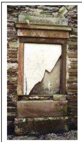
Some gravestones use fitted panels, often in a different type of stone, for the inscriptions or other decoration. Made of thin slabs of stone, these panels can sometimes fall out or crack and break (Figure 46).
